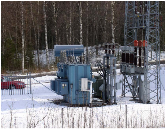
Fig. 1 – 16 MVA, 50 Hz, 3-phase, 55/11 kV, OFWF/OFAF
